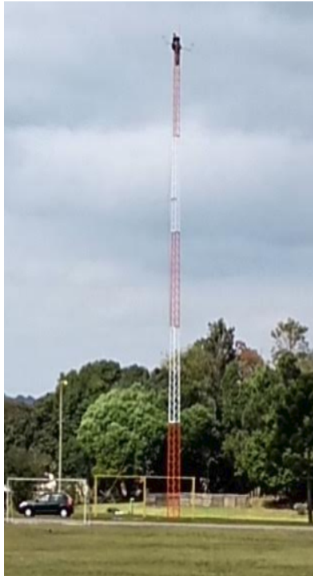
Figura 7 – Torre instalada no campus Neville da UTFPR.
