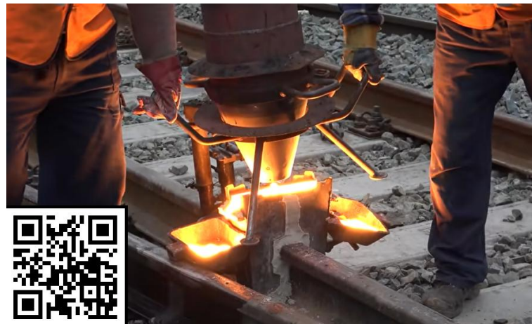
Figure 8 – Continuous rail welding by aluminothermic process on the Serbian Railways in Serbia and Croatia (video).
