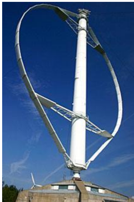
Figura 9 - Turbina Darrieus [18]
