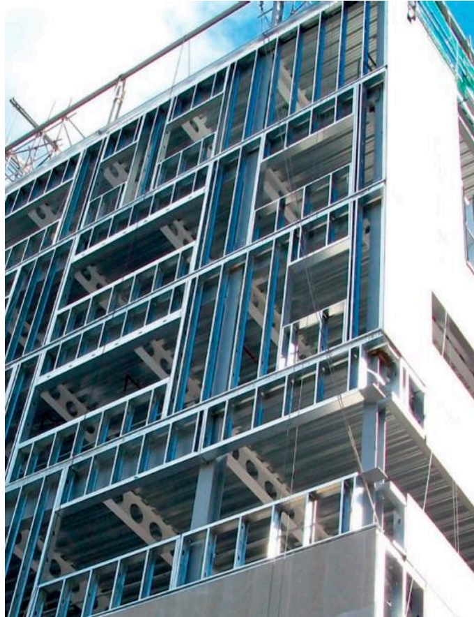
Figure 1.1 – Multi-storey LSF residential building. Adapted from [3].
