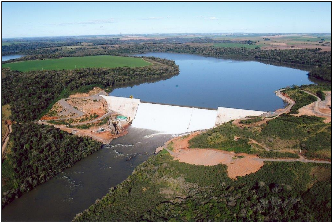
Figura 9 - Barragem UHE Santa Clara ( http://www.panoramio.com/photo/10137558 ).
