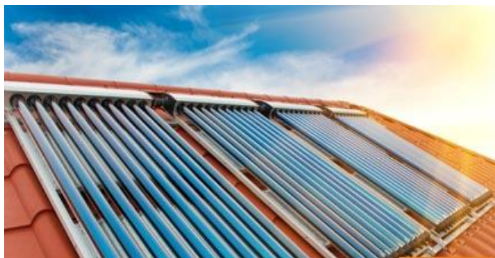
Figura 9- Evacuated Tube Collector.
