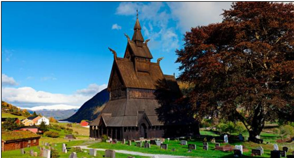
Figura 3 - Hopperstand Stave Church. Fonte:STAVECHURCH (2016)
