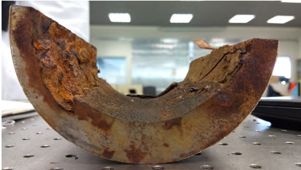
Figure 1 – A Corroded half pipe that was removed of operation for analysis.
