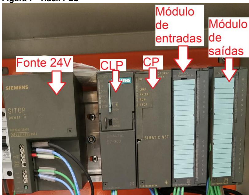
Figura 7 - Rack PLC
