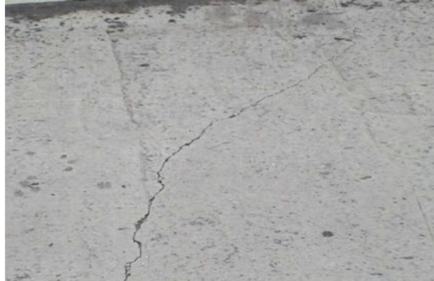
Figura 69 – Fissura diagonal
