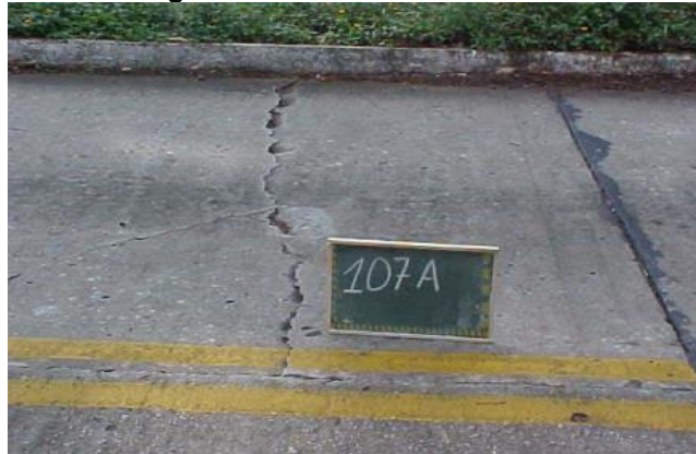
Figura 67 – Fissura transversal
