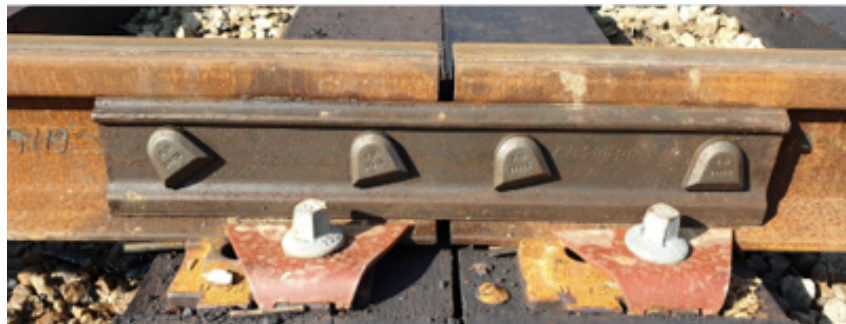
Figure 6 – Fishplate joint
