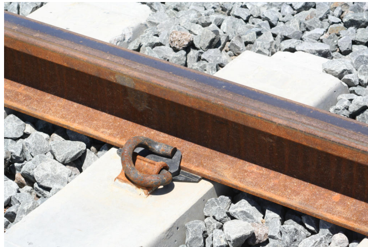
Figure 5 – Elastic Pandrol fastening
